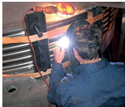
Installation of a clamshell metal expansion joint.
