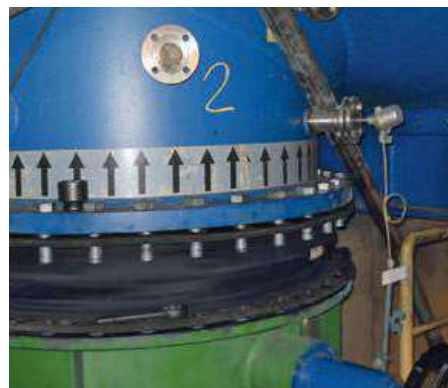
Installation of KE® Rubber Expansion Joint.
