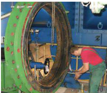
Preparation for installation of KE® Rubber Expansion Joint.
